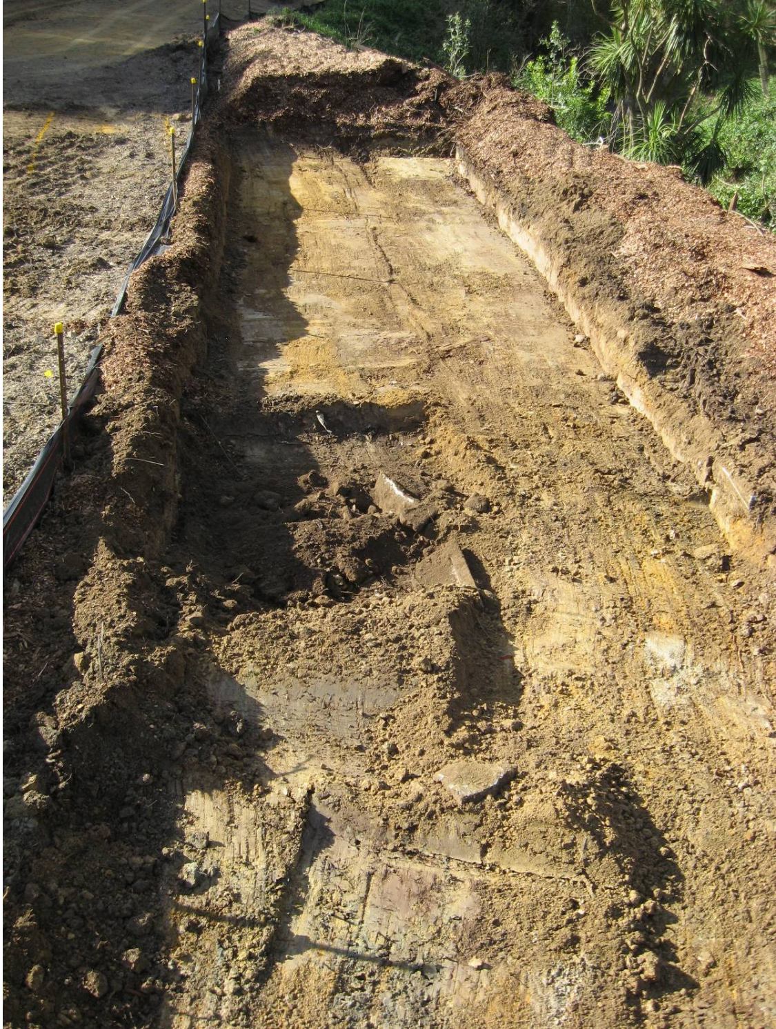
Fig. 10. The silt trap below the road line and by the stream. The only area of intact subsoil is upper left, the rest of the surface is land fill including rubbish, concrete and soil.
