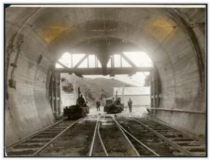
Figure 13: Looking out the No.2 tunnel towards Glenside, as the tunnel is completed in 1933. Evening Post Collection, Ref: PAColl-9150-08, ATL.
