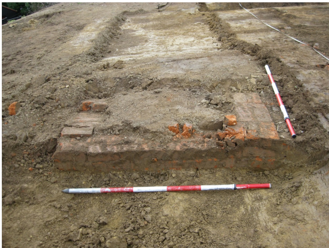
Fig. 13. Chimney/coal range placed-brick foundation, view to south-west.
