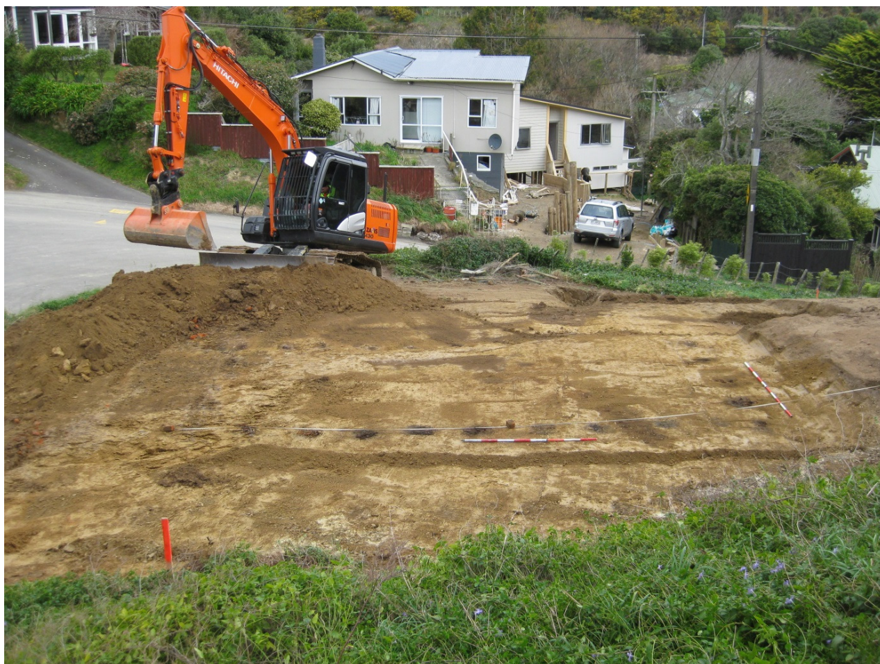
Fig. 15. Last phases of controlled excavation, central and south-west elevation pile holes.
