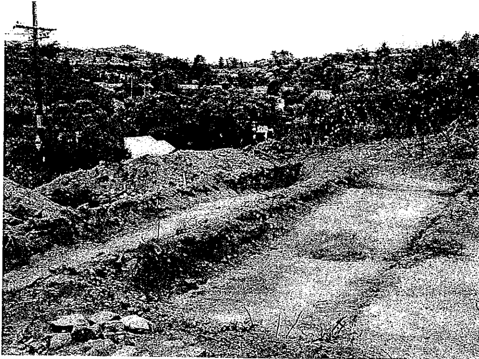
Figure 1: Trenches on terrace, stone and brick mound (bottom left).
