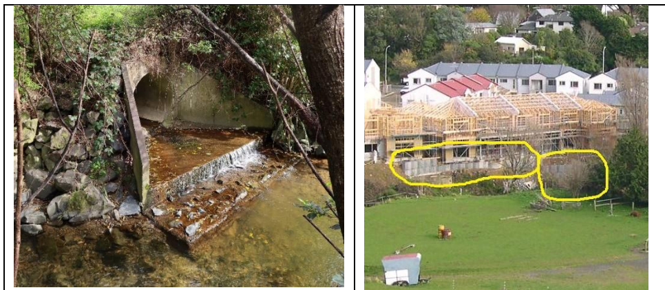
Figure 5. Stream outflow beneath Monterey and detail of Monterey foundation blocks.
