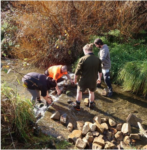
Weir 2 Fish passage construction in Glenside Reserve. 29/06/2023.
