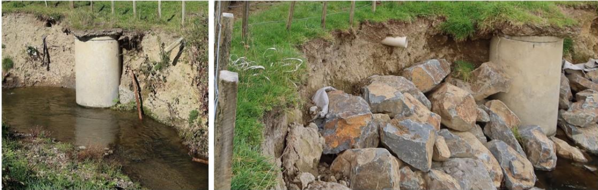
Sewage pipe and bank erosion stabilising 2023. Photo: Claire Bibby
