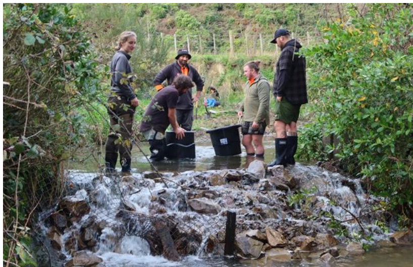
Weir 3 Fish passage construction in Glenside Reserve. 22/06/2023.
