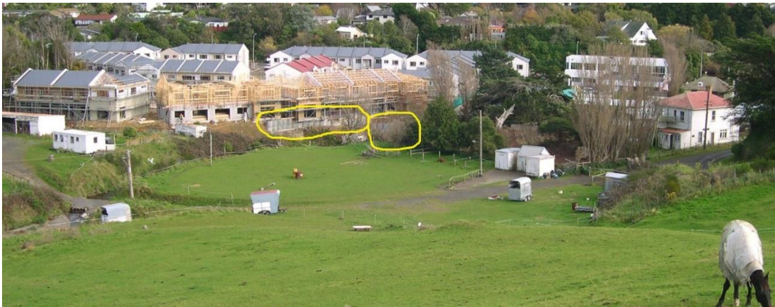
Figure 4. Monterey apartment foundations in the stream bank, 2004.
